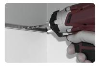
Hold U-channel in required position and drill pilot holes through the channel and into your liner/tiles. A small amount of silicone can be applied to holes and along the length of the U-channel to improve water tightness prior to screwing bracket on.
